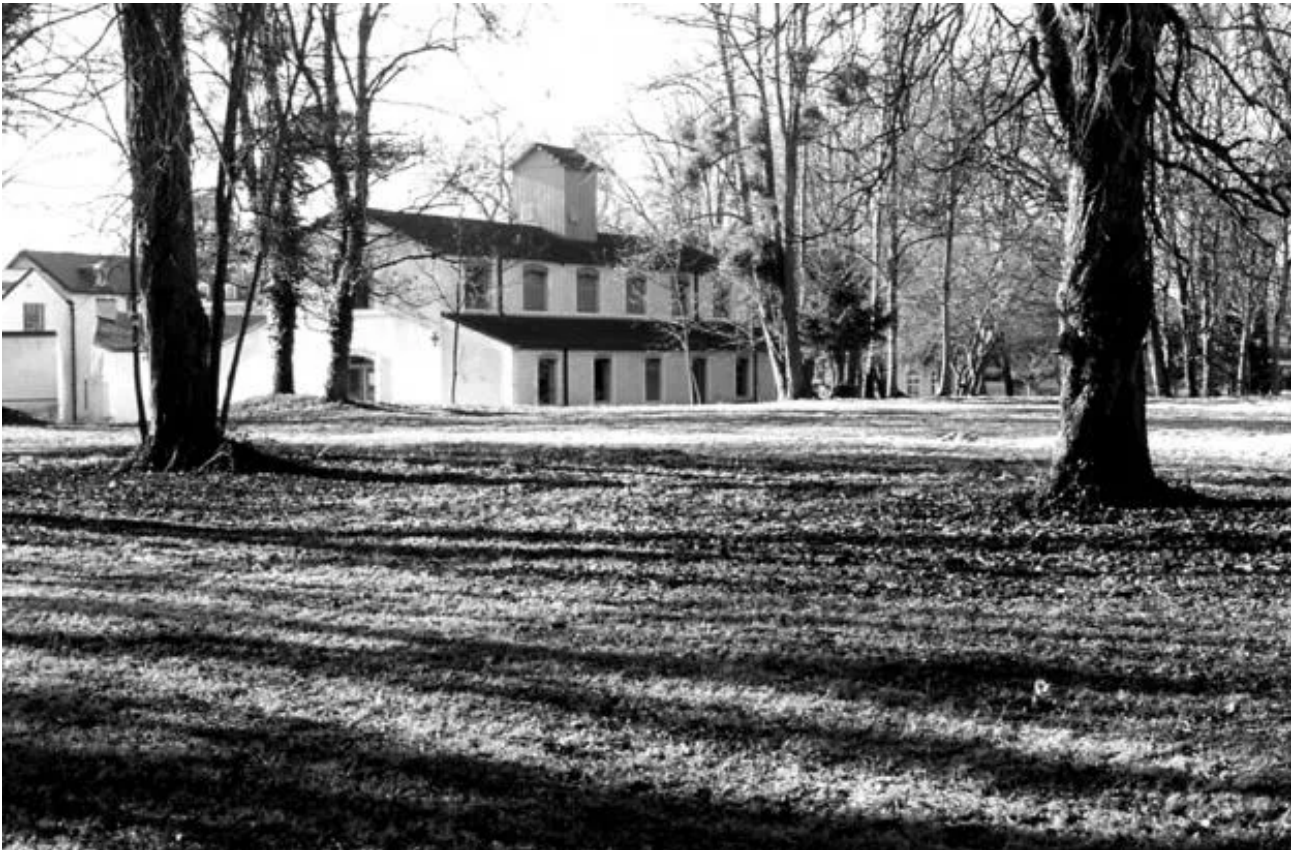
The old bottling factory renovated to house the art center in the departmental park.
